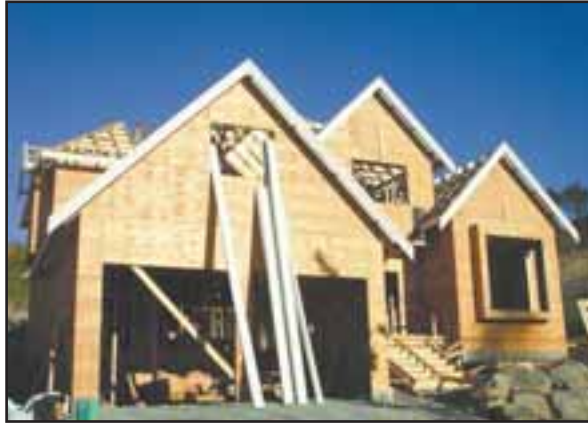
Above, this house shows RealTrim fascia boards during the framing stage.
