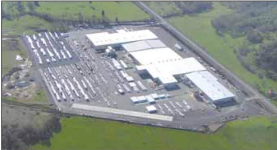
Roseburg's Engineered Wood Products (EWP) plant is one of North America's largest facilities producing RFPI Joists with laminated veneer lumber (LVL) and solid-sawn flange, and RigidLam LVL. The plant covers nearly 70 acres, with over 750,000 square feet of manufacturing space.
