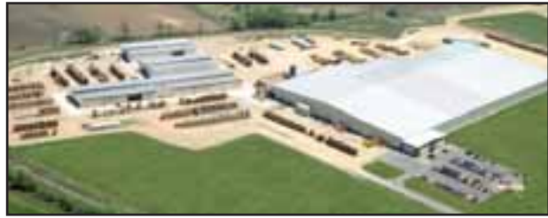
Wolf River Lumber's 55-acre manufacturing facility located in New London, Wis.
