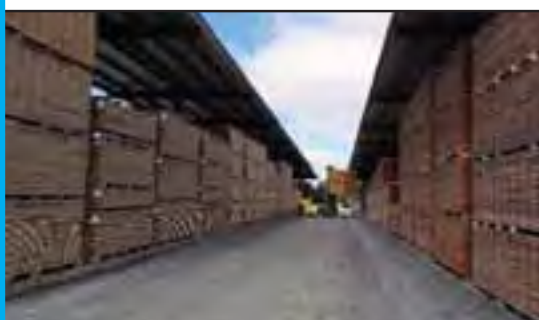
Covered air drying facilities and concentration yard in W. Springfield, N.H.
