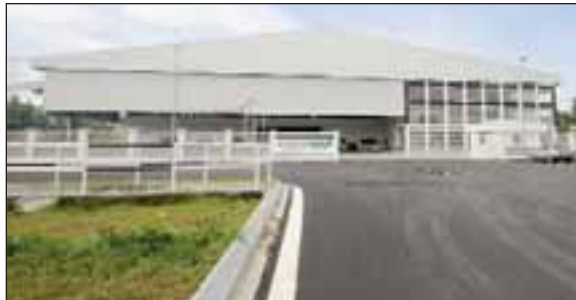
Another Hup Chong facility handcrafts products in this 120,000-square-foot facility.
