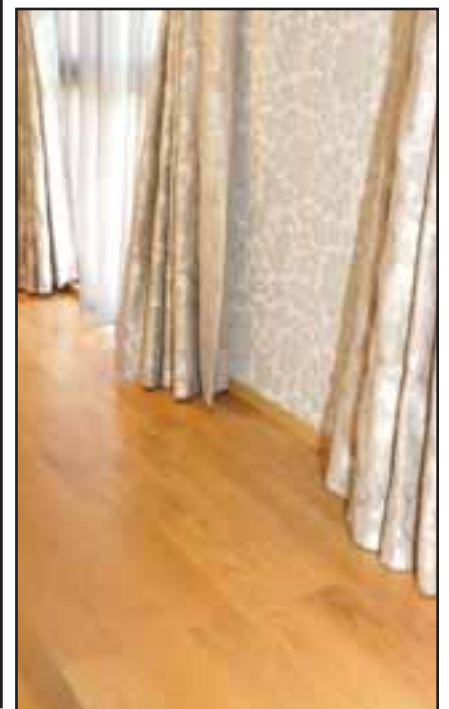
Armany installed this American White Oak flooring and skirting.
