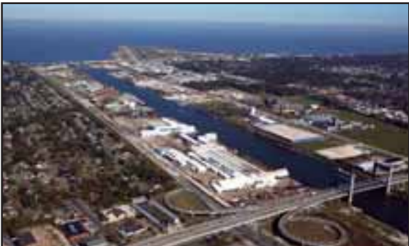
Trinity's vessels, which are constructed at the company's New Orleans and Gulfport shipyards, sell for an average of $30 million.
