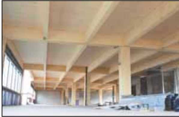
The interior construction of the Fondation building.
