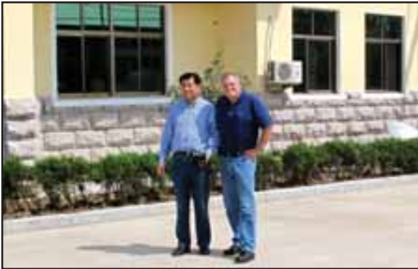
TigerPLY's newest mill and research and development facility that came online in September 2009.
