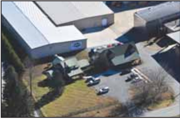
This is an aerial view of facilities at Oaks Unlimited.
