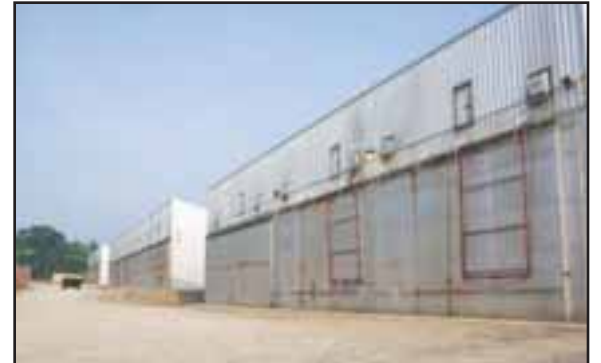
With 12 Nyle dehumidification kilns, Kuhns Bros. Lumber Co. has over 750,000 board feet of drying capacity.
