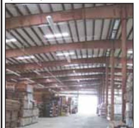
Inside Robinson Lumber Co., Inc.'s new warehouse, the 72,000 square-foot building includes a covered loading and unloading area for flatbeds, four container-loading docks and a mechanical line for grading and sorting lumber.
