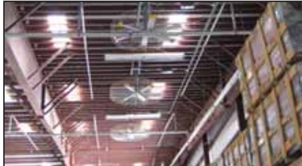
With an area designated specifically for exotic flooring, special fans are in place to provide extra air movement for increased quality of flooring storage.
