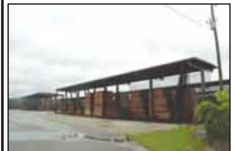
This is a view of a couple of the company's T-Sheds.
