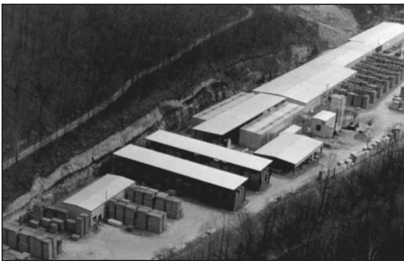
GILCO's dry kiln facility in Roderfield, WV
