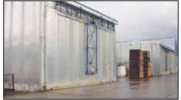
Three of the Bingaman & Son's dry kilns are pictured. The Clarendon location boasts over 3 million board feet of kiln- and air-dried lumber inventory.
