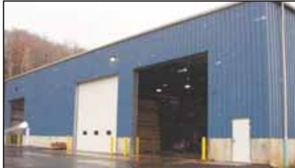
The company recently added a 30,500-square-foot steel building to install a green line and sticking line.
