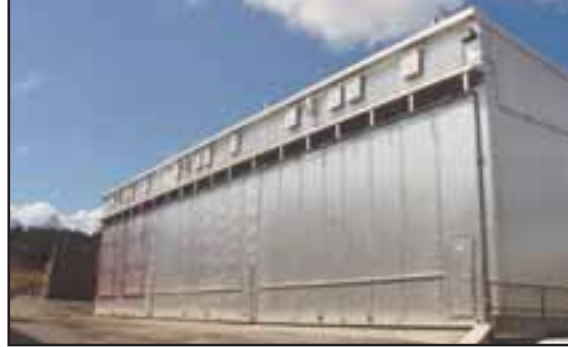
The facility in Liberty is equipped with nine conventional dry kilns manufactured by SII Dry Kilns.
