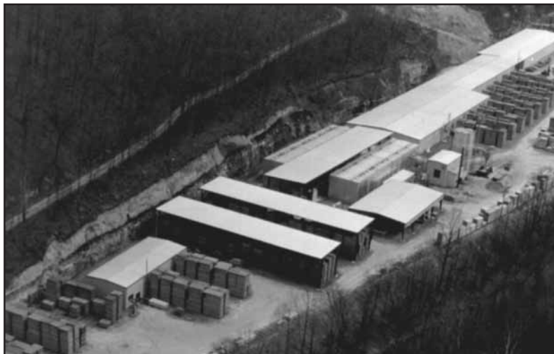
GILCO's dry kiln facility in Roderfield, WV
