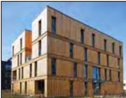
Cross-laminated Timbers were utilized in this structure
