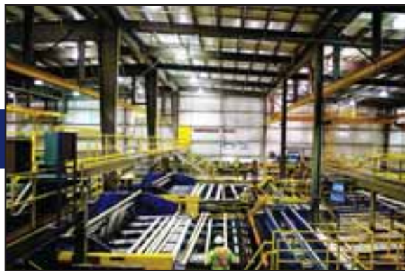
The Adams Lake mill, in the BC Southern Interior was rebuilt in 2012.
