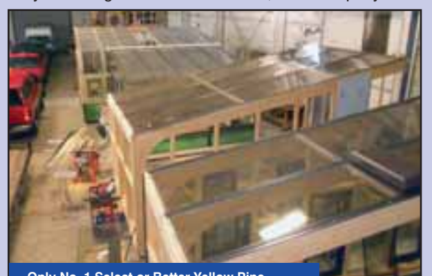
Only No. 1 Select or Better Yellow Pine 2X4’s are used to build frames.
