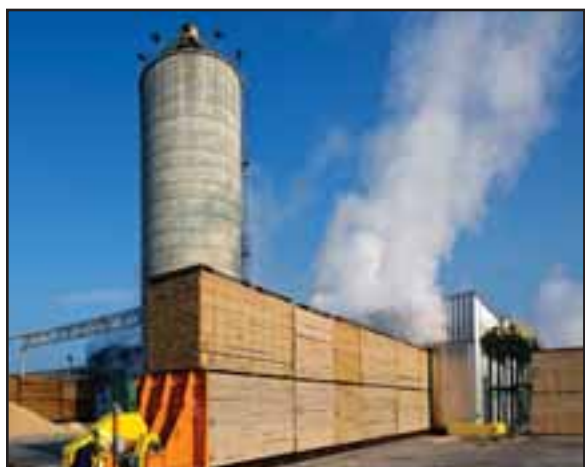
Interfor has purchased six mills in Georgia over the past year, making it the largest lumber company in the state of Georgia. The Swainsboro kiln was rebuilt in 2013.
