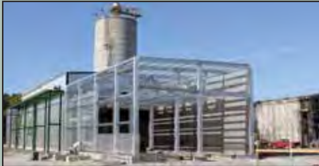
A new kiln under construction at Interfor's Swainsboro, GA, facility.
