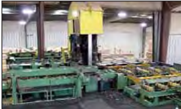
Lumber going through a Corley linebar resaw system.
