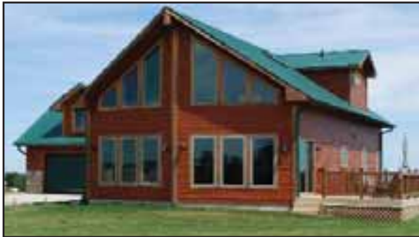
To build an average of 135 homes annually, Heritage Homes procures about 500,000 board feet of kiln-dried lumber.
