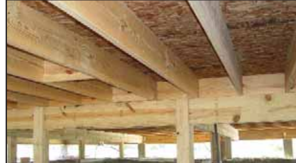
The superior strength properties of Southern Pine lumber make it ideal for raised floor construction.
