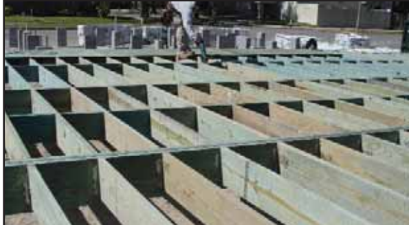
Building a home on a raised wood floor adds a third more lumber to the typical framing package.
