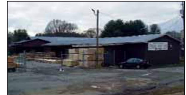
North Georgia Truss operates out of 3 buildings, the 11,000 square foot press room which houses the main Mitek saw and roof truss production line, the 8,000 square foot floor truss production room, and the 5,000 square foot main office and storage building. Pictured is the production facility.
