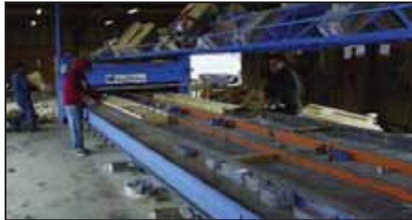
The floor group members at various stages of floor truss assembly in the 8,000 square foot floor truss production room.
