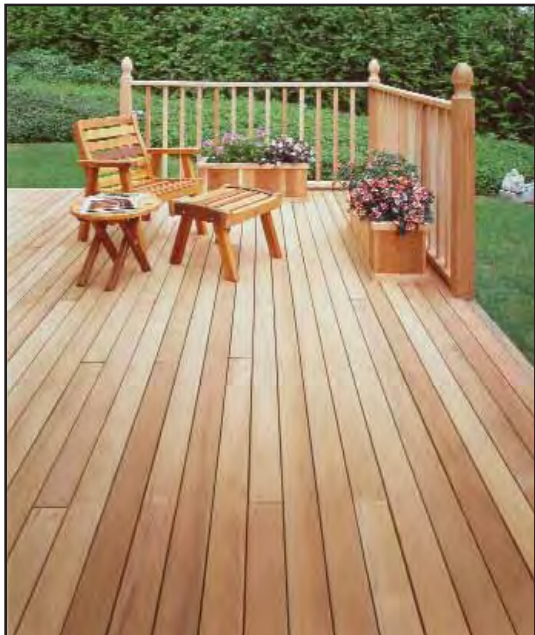
Wood decking is a board-type product horizontally applied in a load-carrying capacity and as the final surfacing for an outdoor flat surface attached to a house and typically elevated above the ground.
