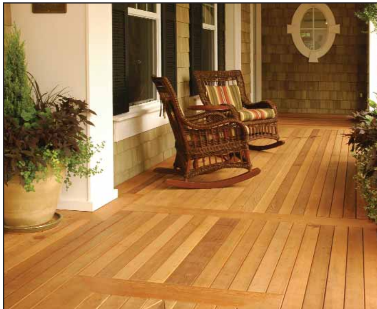
Wood decking is a board-type product horizontally applied in a load-carrying capacity and as the final surfacing for an outdoor flat surface attached to a house and typically elevated above the ground.
