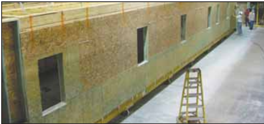
A module for a two-story home is built on the assembly line at the Indiana Building Systems plant in Middlebury, Ind.
