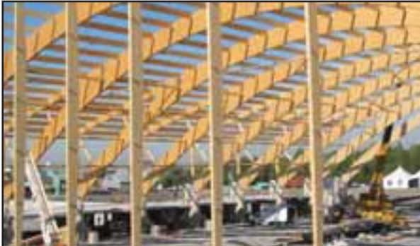
Nordic's Enviro=Lam used here in the construction of a sports complex. This soccer stadium features 210-foot clearspan glulam arches.
