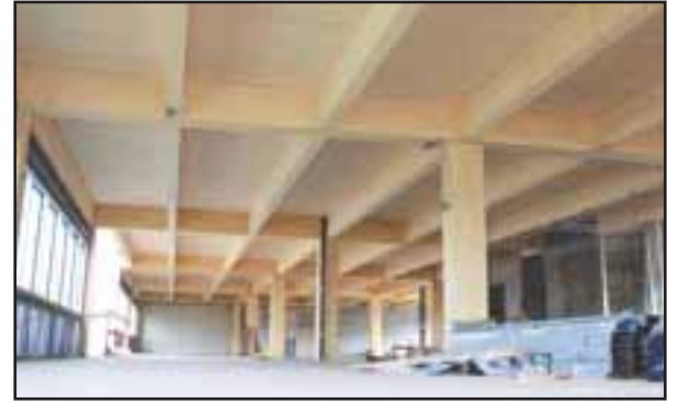
The interior construction of the Fondation building.
