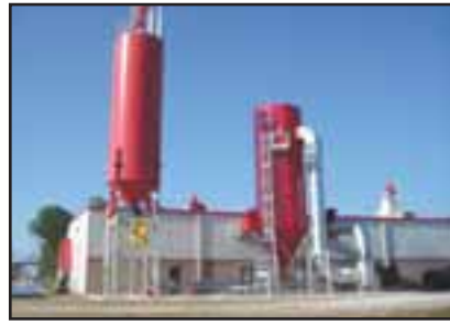
Imperial Systems Converted Wood Biomass Power Plant
