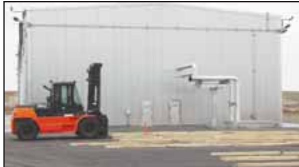
This photo shows the SII side-loading dry kilns that utilize 8-foot-wide lumber bundles, providing superior air flow and even drying.
