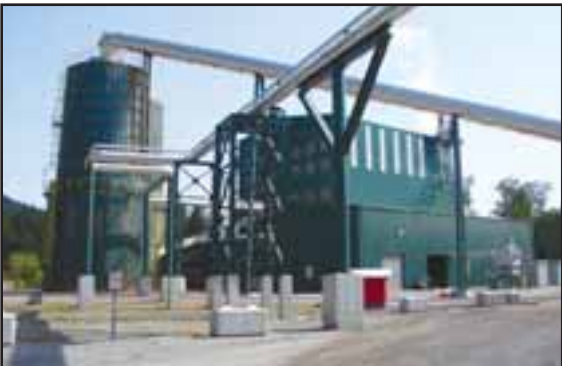
Mill byproducts fuel a new cogeneration plant that heats the Darrington mill's dry kilns and generates electricity, which is sold to the local PUD.
