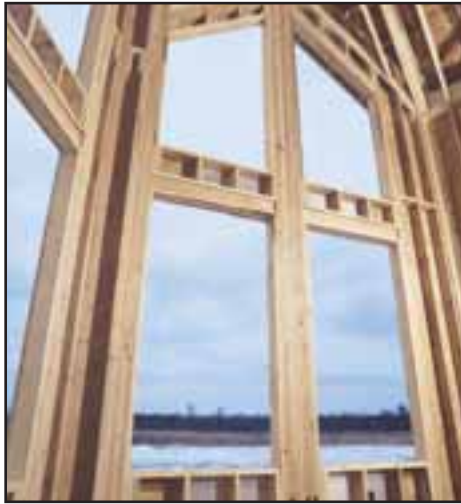
As homeowners demand tall walls in their kitchens and living rooms, Rosboro has responded by offering lightweight and load-wrapped glulam columns. The columns can be easily nailed, bolted and cut, eliminating the need for nailing and bolting in "built-up" columns.
