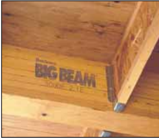
Rosboro's Big Beam® combines strength, stability and versatility, making it a popular product among builders. Big Beam is made in typical I-Joist depths of 9 1/2-inch, 11 7/8-inch, 14-inch, 16-inch and 18-inch, and is sized to match framing widths of 3-1/2-inch, 5-7/16-inch and 7-inch.
