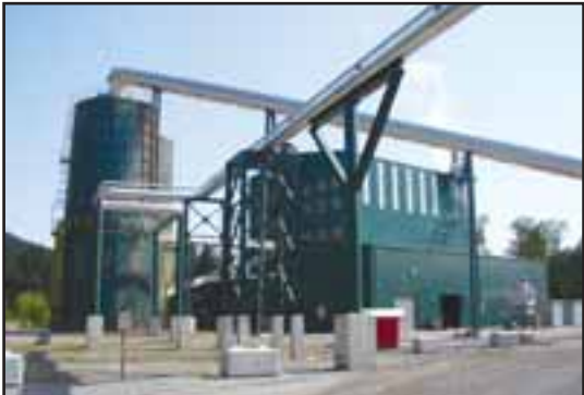
Mill byproducts fuel a new cogeneration plant that heats the Darrington mill's dry kilns and generates electricity, which is sold to the local PUD.
