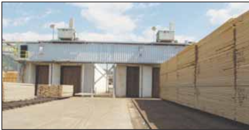
In recent years, J D Lumber added four 120-foot-long double-track dry kilns that can handle 1 million feet of lumber.
