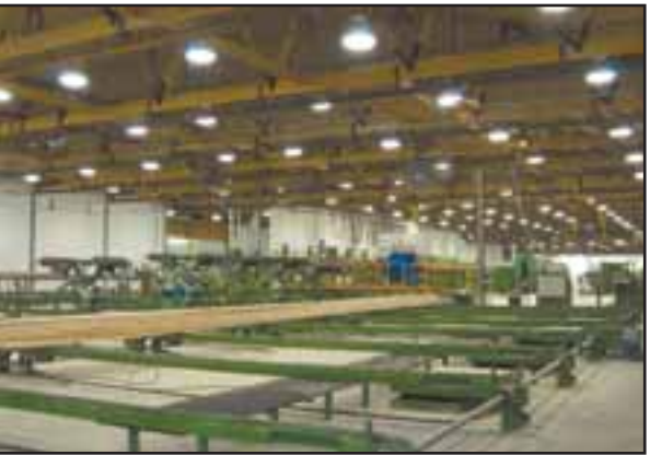
QB Corp. recently completed an expansion project, which added two automated presses and another high-speed finger jointer. An additional curve rack was also installed to reduce lead times.
