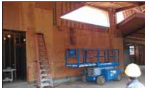
The Pico Branch library is shown under construction using Roseburg sheathing.
