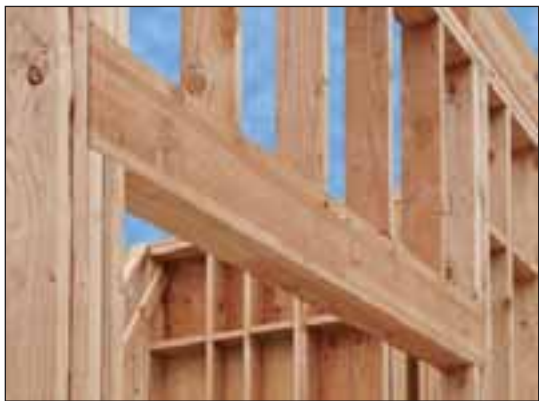
Pictured is Rosboro's X-Beam frames installed flush against framing.
