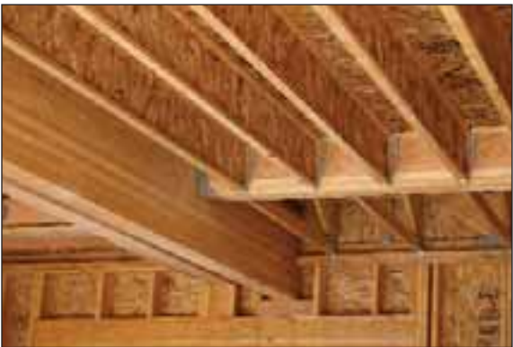
Shown here is how the company's X-Beam matches the I-joist in depth.
