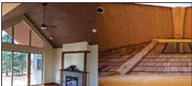
A significant portion of Woodtone's RealWood™ product volume is dedicated to the company's RealSoffit™, pictured here, which is an end matched tongue and groove v-joint wall and ceiling paneling product.
