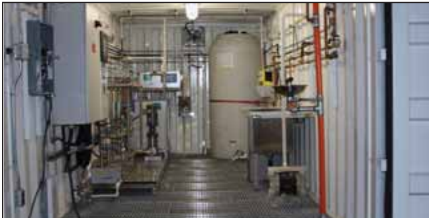
The Diaplex™ 100 TurnKEY makedown system is pictured.
