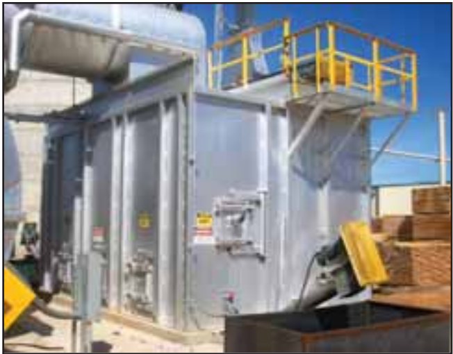
USNR's new 8-grate Green Fuel Burner produces approximately 40MM BTUs of heat per hour, and is proven to keep high value lumber in the kiln remarkably clean and free from ash.
