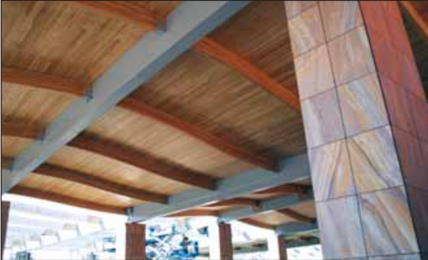
Laminated wood roof decking is for architectural applications where the beauty and ambience of a natural wood ceiling is an important element of the architectural style.
