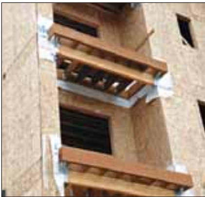
The Rosboro X-Beam is manufactured to match standard framing and is available in conventional and I-Joist depths.
