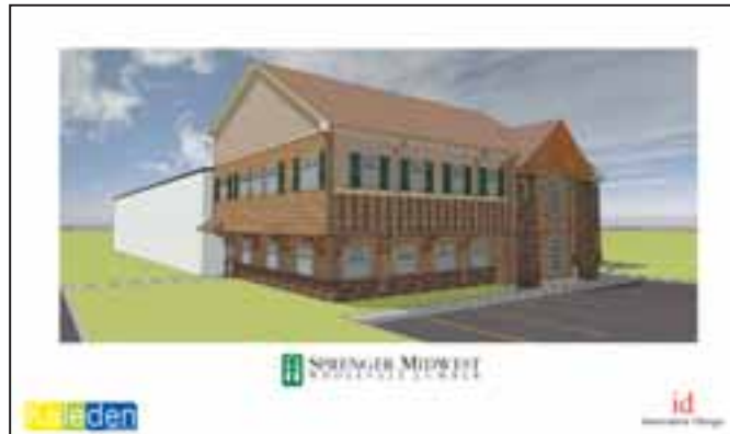
Sprenger Midwest recently completed construction of a new office building at their main location in Sioux Falls, which doubles their office space.
