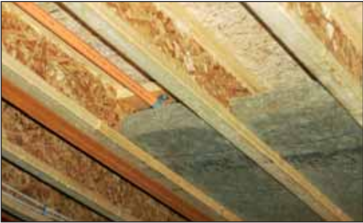
Boise Cascade BCI(R) or AJS(R) I-joists team with mineral wool insulation to insulate better and suppress residential fires for longer periods of time.
