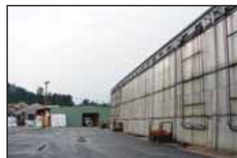
King Forest's dry kilns and storage buildings.
