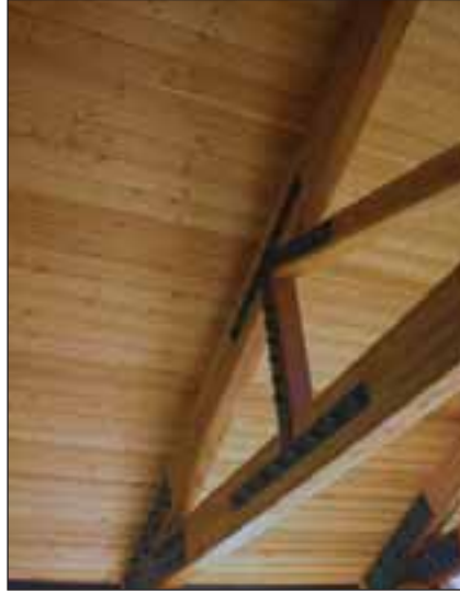
Among the many popular products manufactured by Disdero Lumber Co. of Clackamas, OR, is lock-deck/roof decking. This structurally engineered product consists of two to five kiln-dried lumber laminations bonded together with an exterior waterproof adhesive to form glue-laminated decking.
