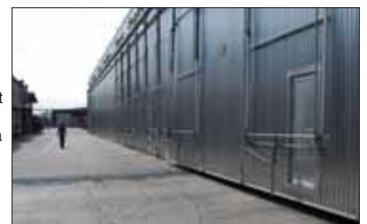
Pictured are recently installed dry kilns at Cersosimo Lumber Co. Inc.
