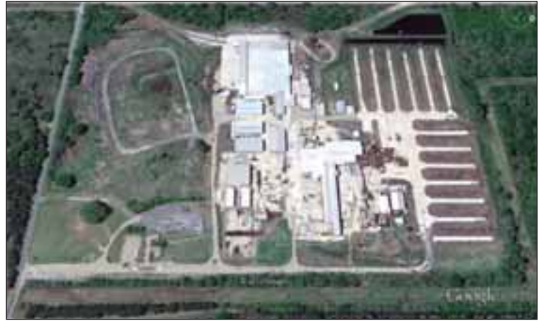
Idaho Timber began the process of refurbishing and extensively upgrading this sawmill in Coushatta, LA, which was previously owned and operated by Hood Industries.
