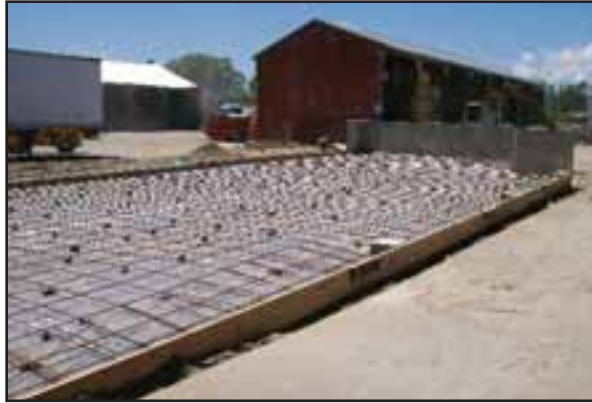
Hancocks new Pittsfield moulder facility under construction.
