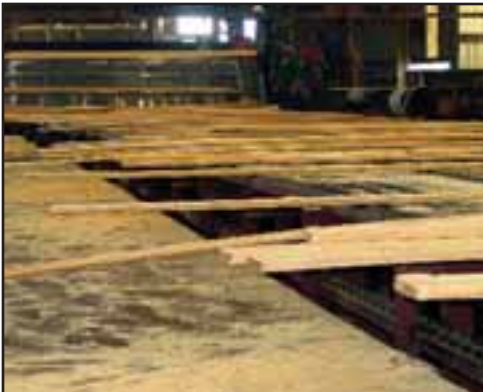
With a fully enclosed facility of over 220,000 square feet of finished lumber storage and loading, Snider prides itself on the clean, dry and dust-free delivery of their finished lumber. The lumber stays under roof and is never exposed to elements once the drying process is complete. Customer trucks are able to load, weigh and tarp inside the massive building. Snider can provide most items for immediate, same-day shipment.
