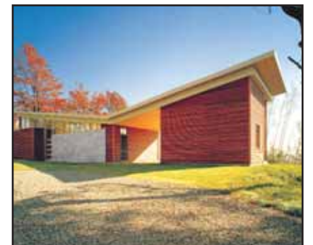
Western Red Cedar siding has a significantly lower environmental footprint than fiber-cement products.
