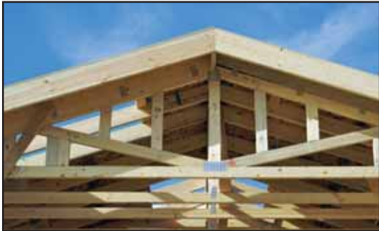
Pictured is Softwood used in roofing.
