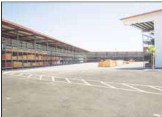
This photo taken at Big Creek Lumber in Atwater, Calif., shows a Powerbin automated lumber storage rack supported three-sided shed.
