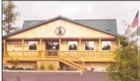
The Washington operations for Mary's River Lumber Co. are located at Montesano, where all facets of manufacturing are performed at one location.
