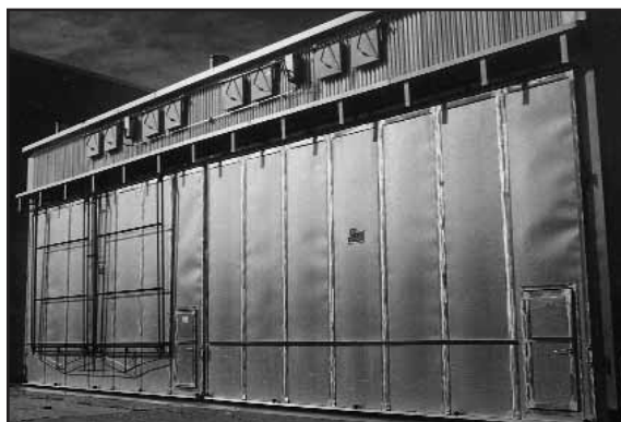
Frontal view of dry kilns.
