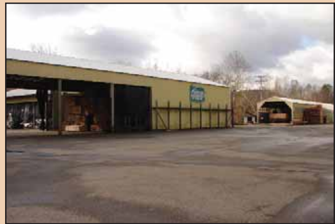
This photo shows lumber being staged for shipment in a storage building on the left, while lumber is being taken off sticks on the right.
