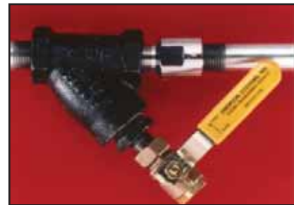
The Enercon assembly used by Yoder includes permanent condensate removal unit, Y-strainer, blowdown valve and nipple.
