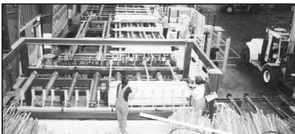
At the new Hardwood concentration yard in West Jefferson, NC, owned by Gus Newton, Brian Becker, and David Blair, the firm installed new lumber handling equipment. Shown here is the new stacker line with the tilt hoist shown towards the top of the picture.
