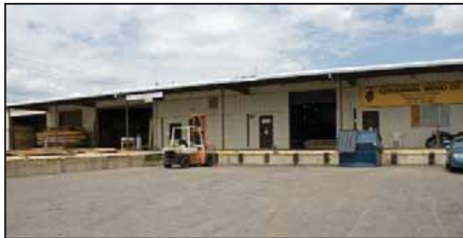
Centennial Wood Company's 20,000 square foot mill shop sits in the middle of their 80,000 square foot yard, giving it plenty of room for expansion.
